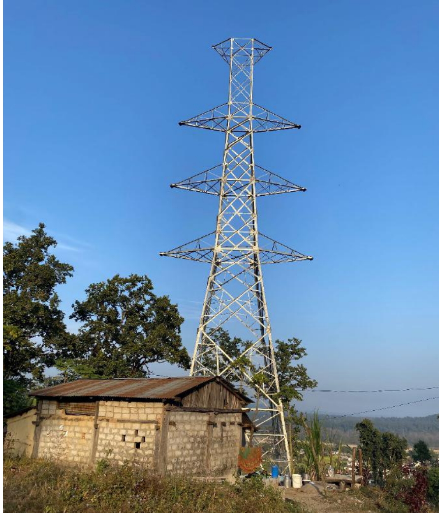
Photo 1. Example of a building (close to tower no. 200) that has to be compensated for and moved
